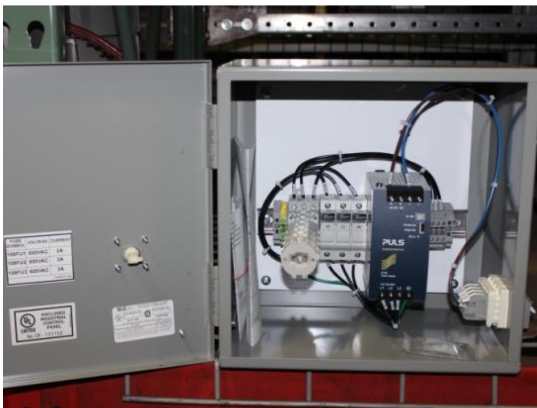
Motor Control Power Supply with Branch Circuit Protection (10A 480 VAC shown)
