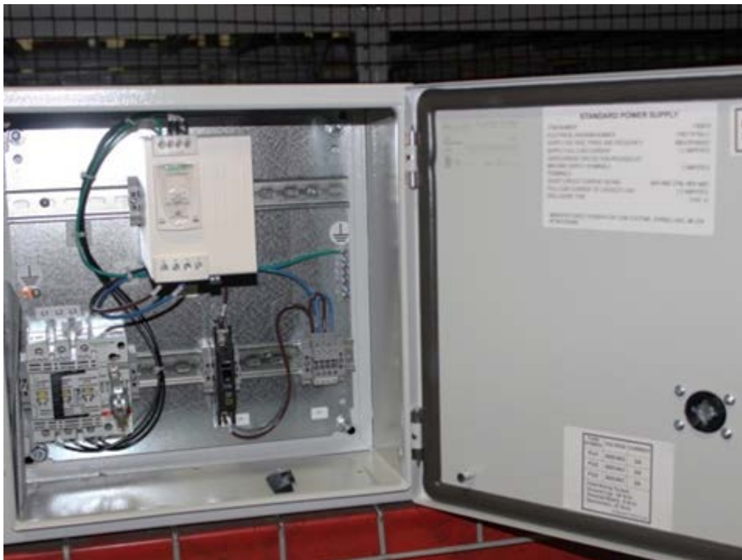
Standard IntelliROL Power Supply with Branch Circuit Protection (20A 480 VAC shown)
