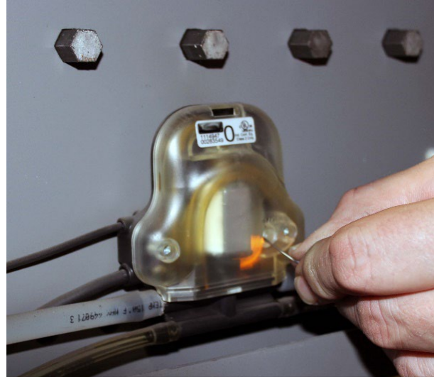
Amber light indicates progressive mode. Toggle Switch (use paper clip to change)
