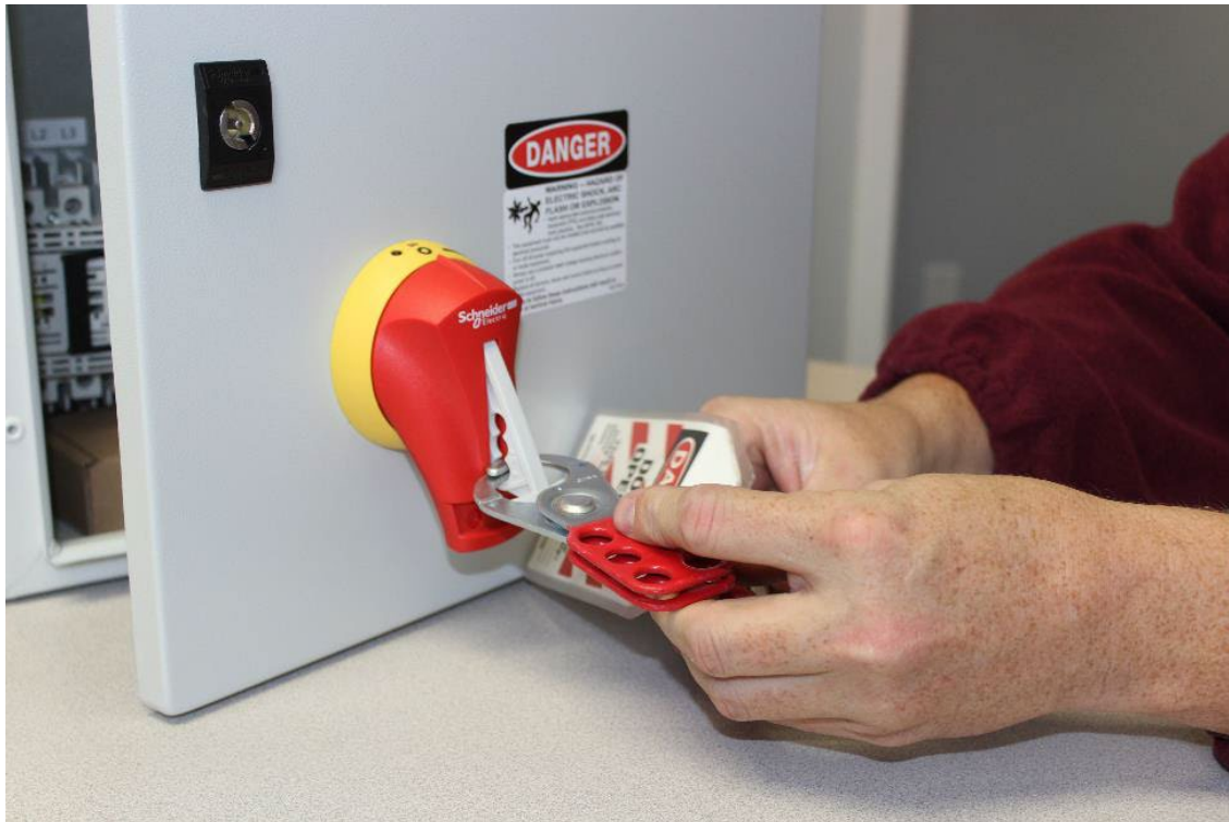
IntelliROL Power Supply Lockable Disconnect Switch
